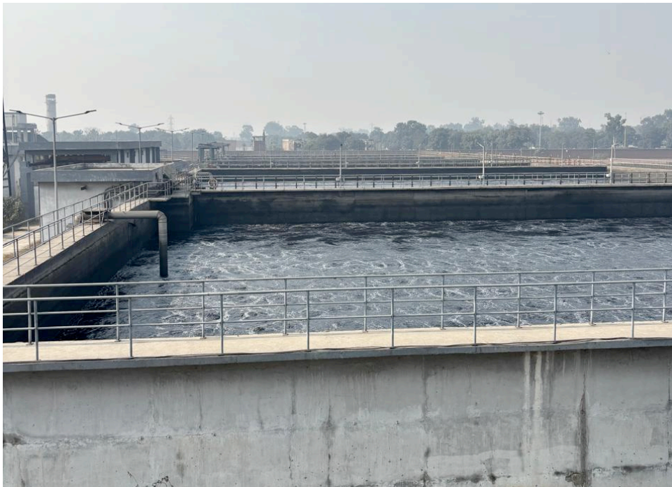
Figure 1: View of 50MLD CETP
